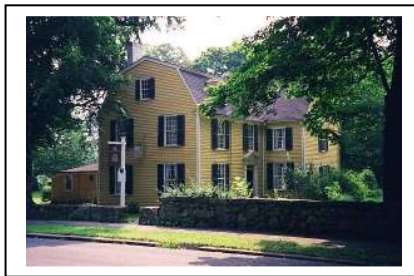
Present Hale House w/ 1745 gambrel addition which replaced the 1695 lean-to & current road location
